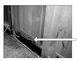
Keyboard Pullout locking Screw (Must be removed)
